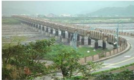
Figure 1. Taiya Bridge View
